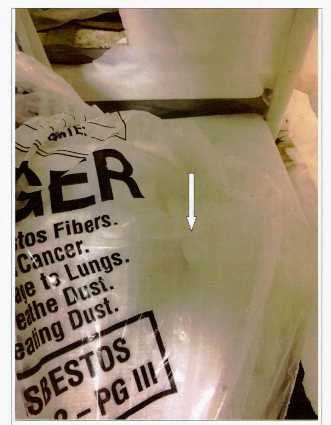
Photo #: 4 Description: A bag pulled from inside containment. According to the on-site supervisor, the generator labels inside the bags were crumpled and unreadable at the time of inspection due to the water inside the bags.
