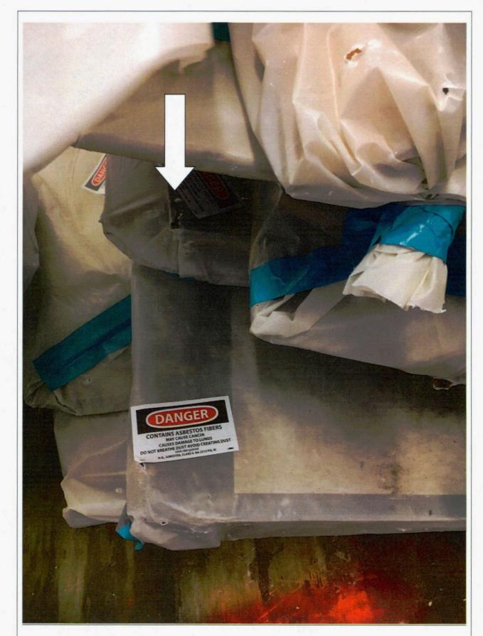
Photo #:  $\underline{3}$  of  $\underline{5}$  Description: "Burrito wrapped" sections of flooring were not wet or leak tight. Holes were visible throughout multiple sections. Generator labels were not present at all.
