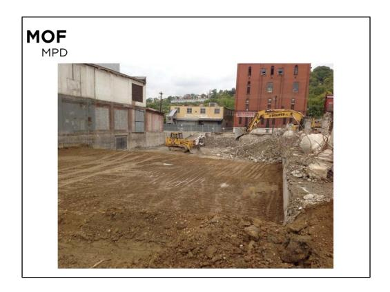
Moving on to the Maintenance and Operations Facility, or M-O-F, work's underway on that at Henry and Race streets. We've already demolished the two buildings there and are working to prep the site for construction. As of this week, foundation work has begun.
