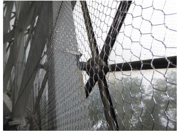
Figure 13. Close-up of netting in Show Dome
