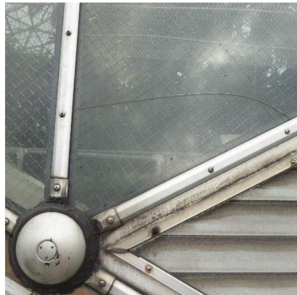
Figure 21. Cracked glass
