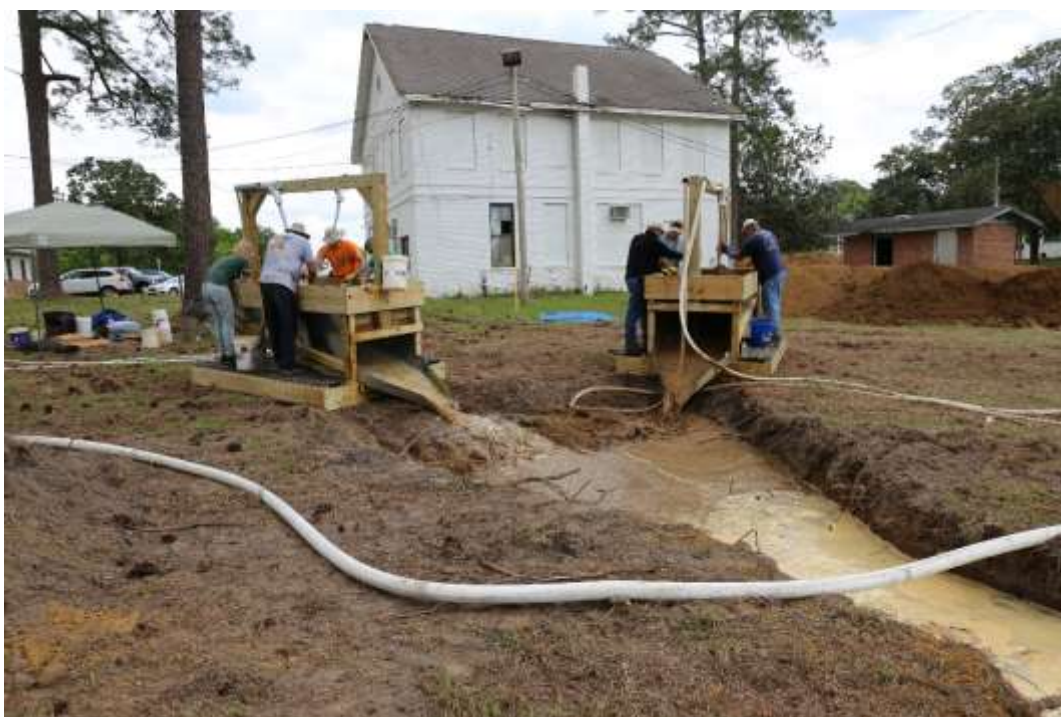
Figure 48. Water and sediment run-off into a slit trench leading to a holding pond to trap the sediment while allowing the water to run off into a natural drainage.
