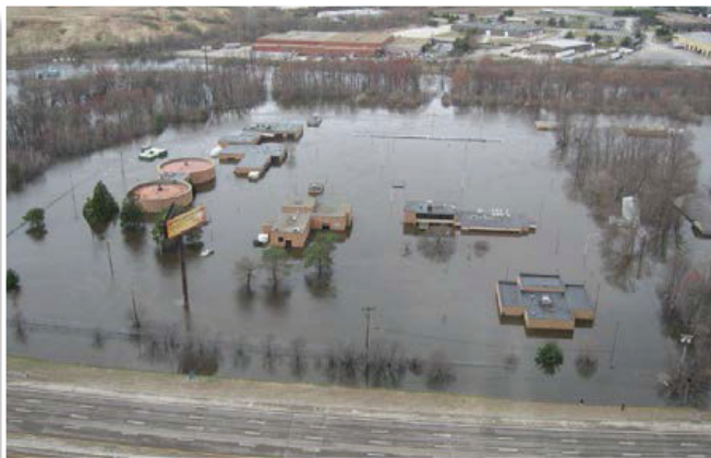
The flooded Warwick wastewater facility sits between the surging Pawtuxet and the closed Interstate 95 during the floods of 2010.
