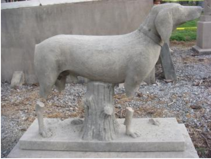
The dog figure was missing parts of his feet. Threaded stainless rods were first epoxied in place to be used as armatures for Jahn mortar.
