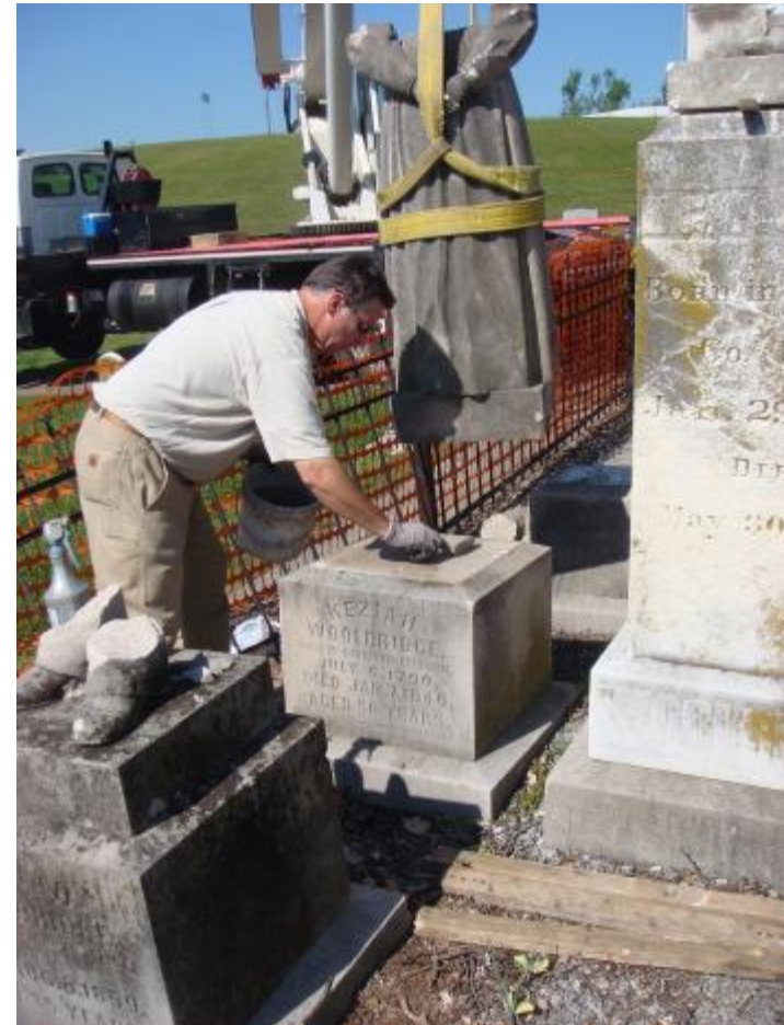
Preparing the setting surfaces and resetting Keziah Wooldridge with 000 mortar..
