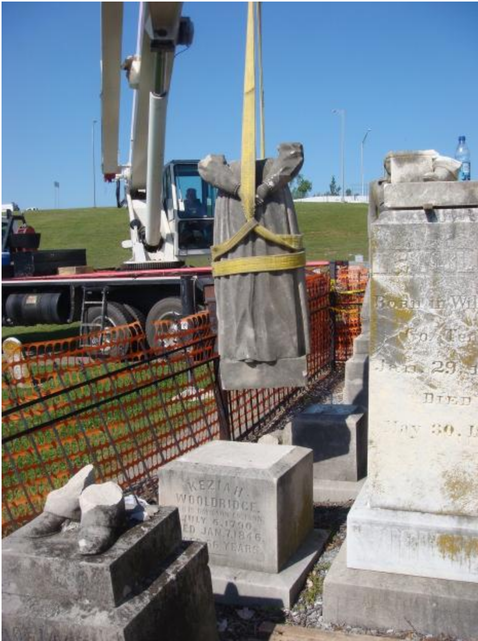
Preparing the setting surfaces and resetting Keziah Wooldridge with 000 mortar..
