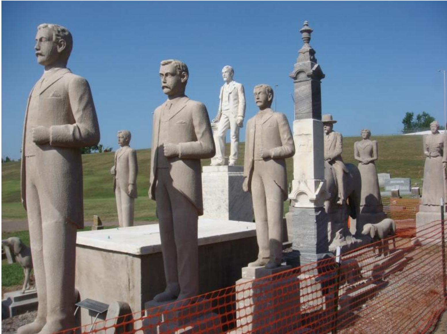
July, 2010. All small cracks filled with 000 pigmented crack filler and larger losses filled with pigmented Jahn restoration mortar
