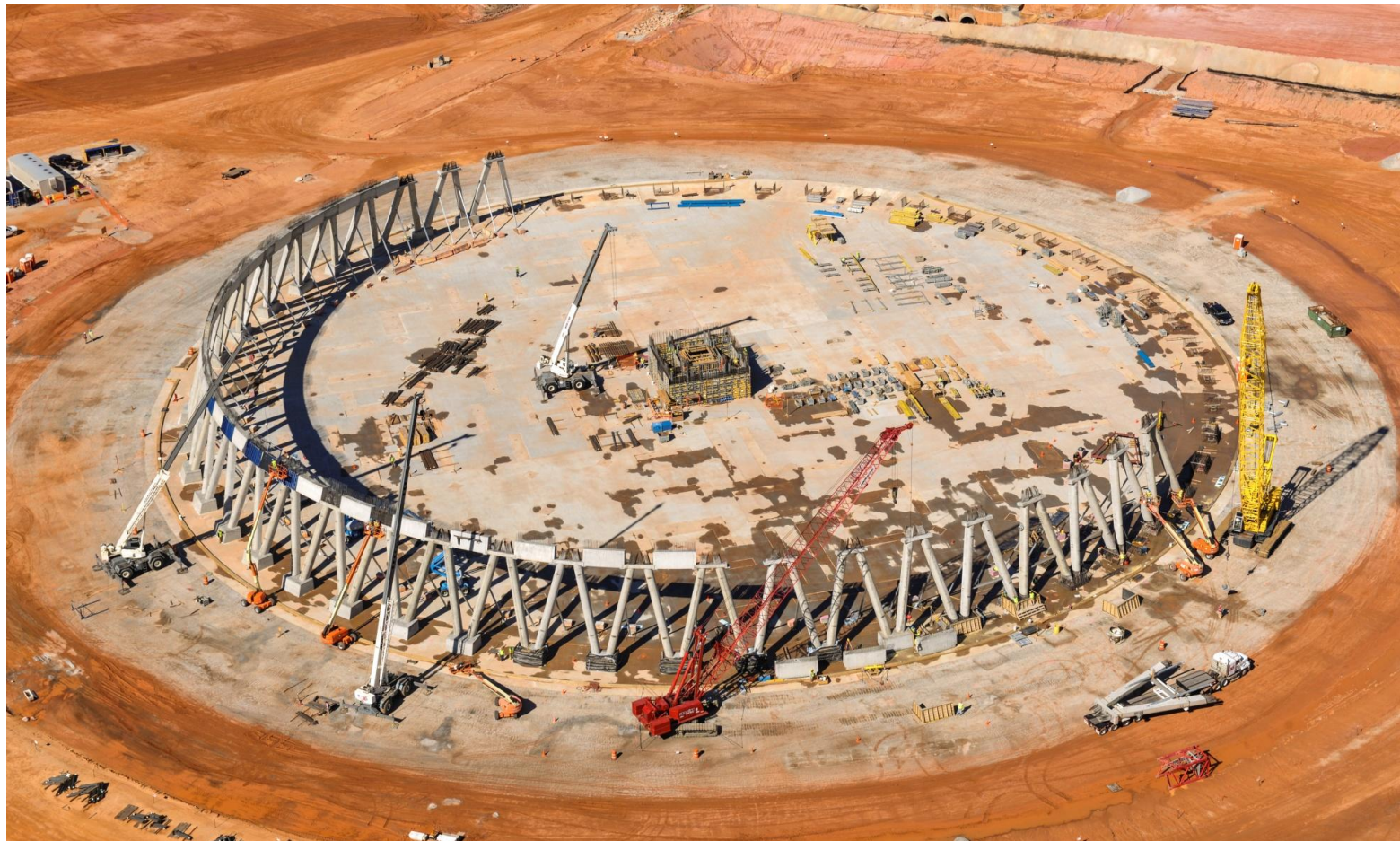
Plant Vogtle Unit 3 cooling tower construction
