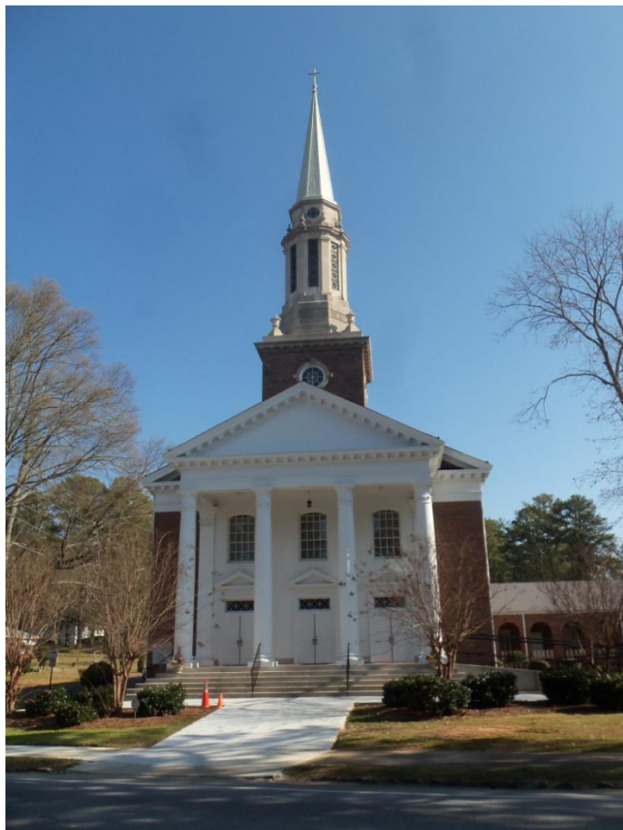
Figure 6. Formerly Audubon Forest United Methodist Church, this building is now used by Hoosier Memorial United Methodist Church. (photo by author)
