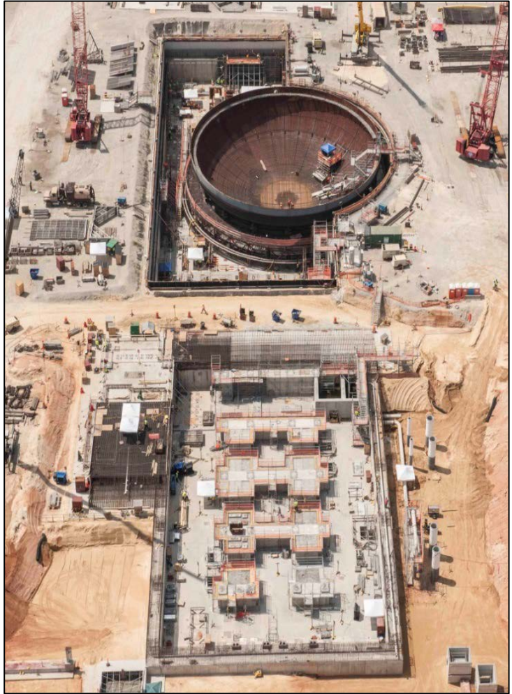
Photo 12 - Unit 4 Nuclear Island and Turbine Island
