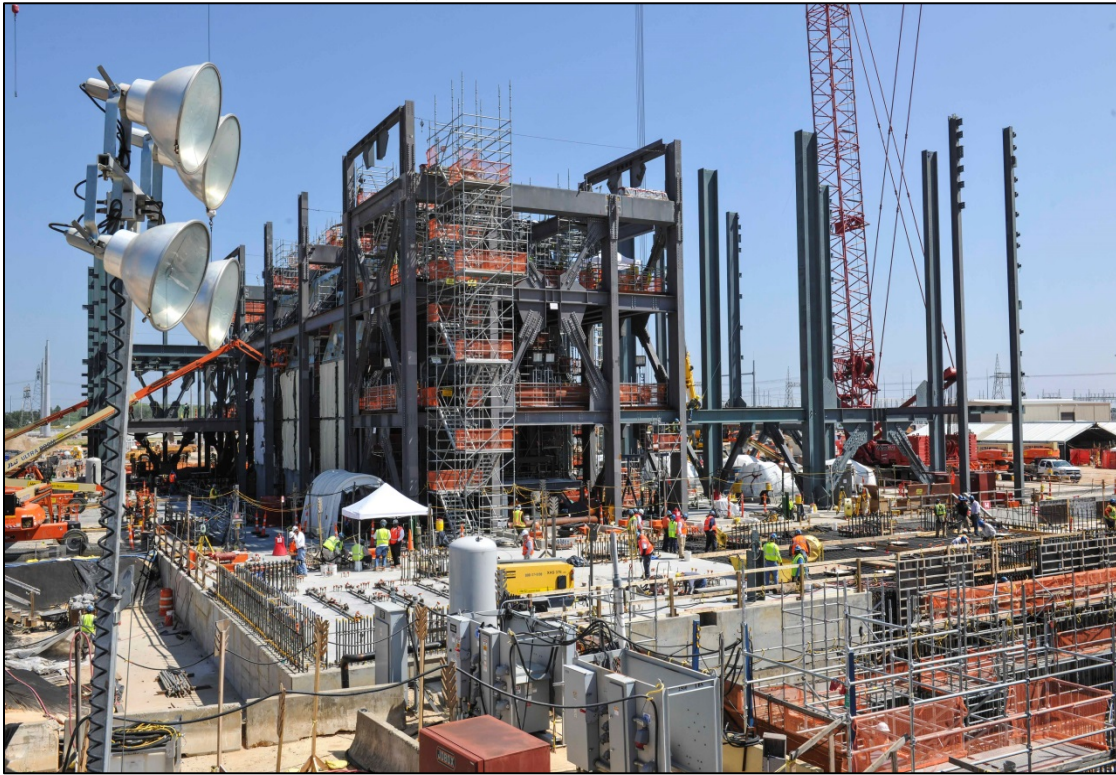
Photo 9 - Unit 3 Turbine Building
