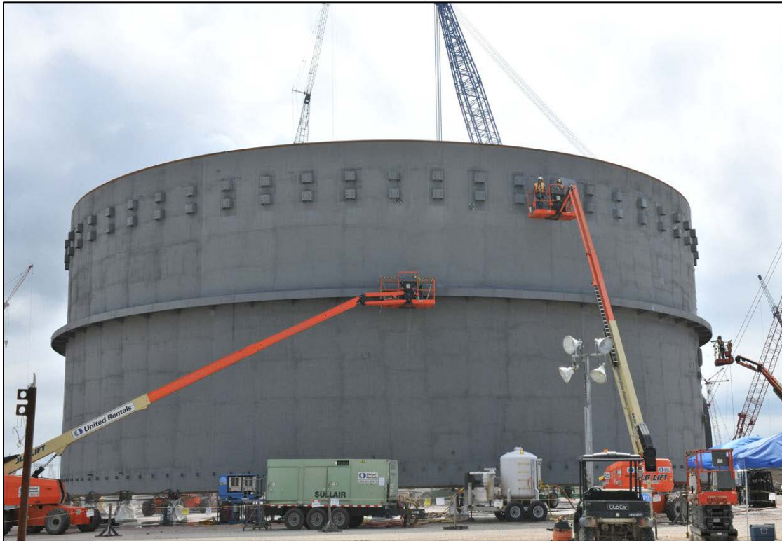
Photo 5 - Unit 3 Containment Vessel Lower Ring Coating Activities
