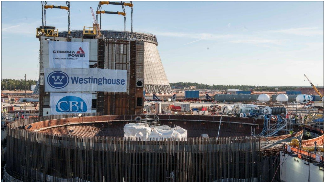
Photo 3 – Unit 3 CA20 Lifted into Nuclear Island
