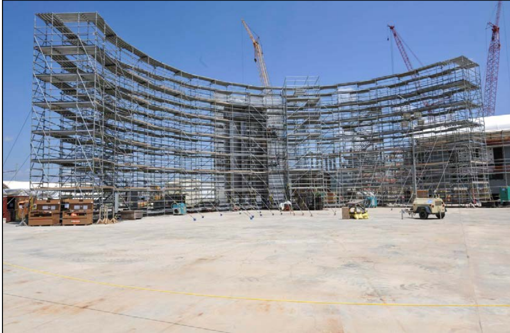
Photo 7 - Unit 3 CA03 Pre-Assembly
