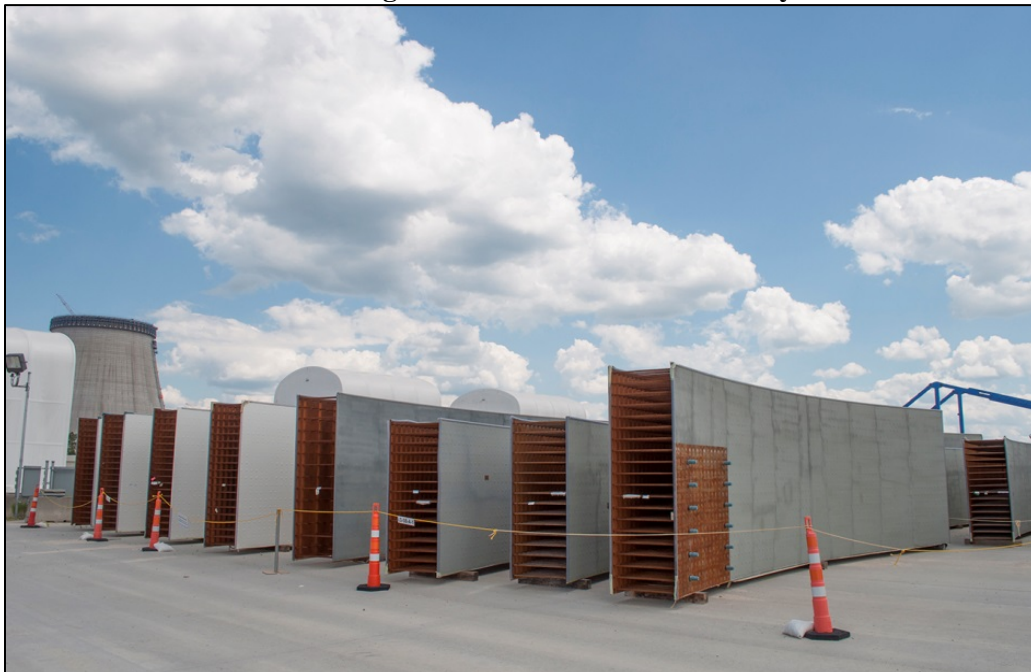
Photo 8 - Unit 3 Shield Building Panels Delivered to the Facility
