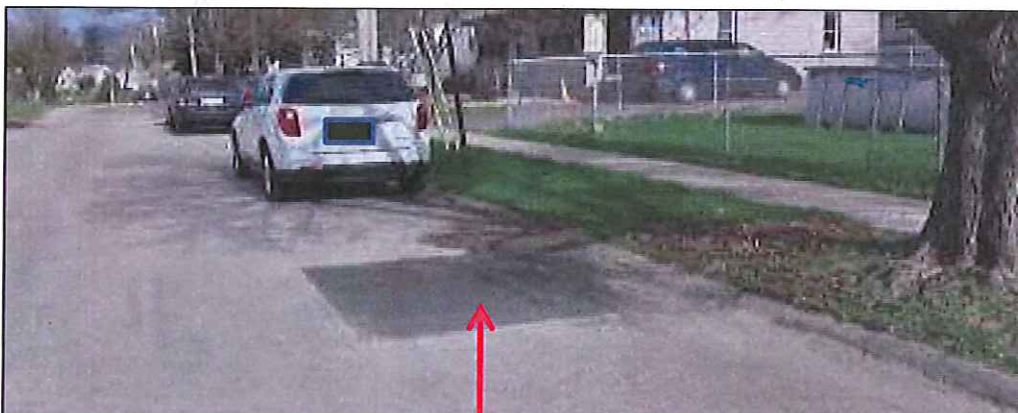
Recent patch (#2) of asphalt along curb next to the parkway where the [redacted] service line runs.
