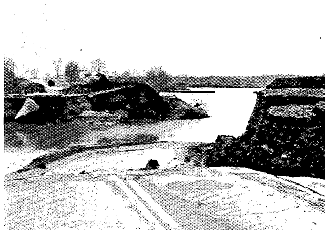
Part of IL Rt. 23 which was washed out when a dike broke. ---Photo by C. Kinas.
