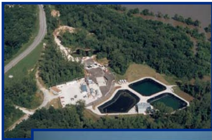
Quarry Looking Northeast; Bulk Waste Removal Completed December 1995
