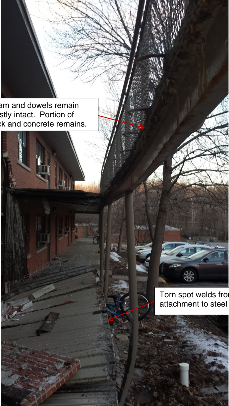
Photo 5: Remaining Front Edge Beam, “J” Dowels, Railing & Torn Fasteners
